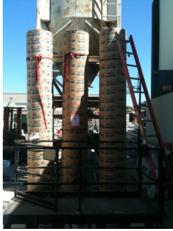
Performing the 10' Sonotubes Stable Flow™ tests on site
